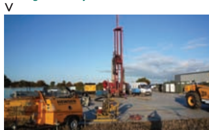
Drilling at Fradley Junction
