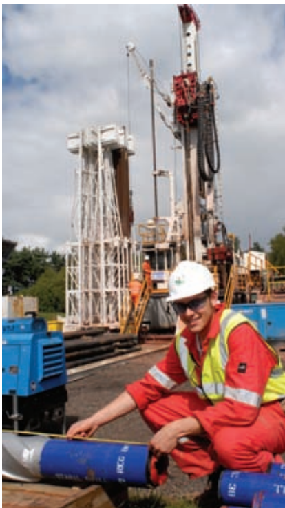
< Drilling operations in Staffordshire
